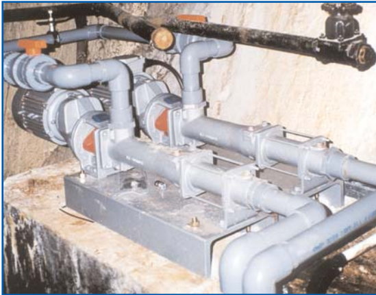
The positive displacement action of these pumps prevents build up of manganese for ground water pumping, resulting in continuous operation
