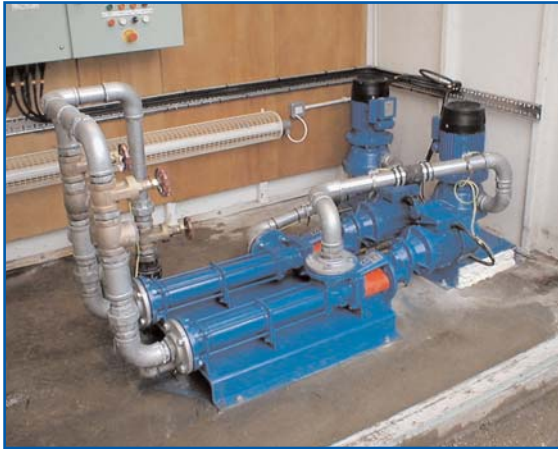
A Mono packaged pumping system comprising pumps and macerators to pump raw sewage
