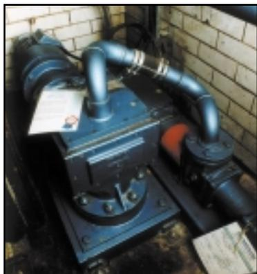
Public toilets, located directly beneath a local tourist information centre, are open 24 hours, but not attended at night. This results in abuse of the drainage system, with drink cans and other items of indiscriminately disposed of waste found in the sump. A compressed air operated sewage ejector system was previously installed but could not cope with this abuse. It required weekly maintenance visits and was extremely noisy.
