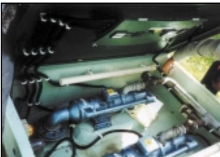
Funded by a £70,000 grant from the National Lottery, a new bowling pavilion has installed a Grifter Packaged Pump Station to transfer all wastewater from the pavilion's services to the main sewerage system over 20m away. Foul and wastewater from the pavilion's washrooms and catering facilities are directed to the Grifter's holding tank, which incorporates float switches. The pump is triggered when the effluent reaches a pre-set level and switches off when the stop level is reached.
