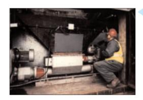
A W064 model installed at a sewage treatment works to control sewage odours, caused by a belt press feeding dewatered sludge cake directly onto an open-air conveyor and into an open skip for disposal. The cast iron W064, with an integral bridge breaker fitted as an option, delivers the sludge cake at the required rate of 2.5m³/h and pressures of up to 12 bar. It operates eight hours per day, six days a week and daily fills up the four enclosed skips with sludge cake.
